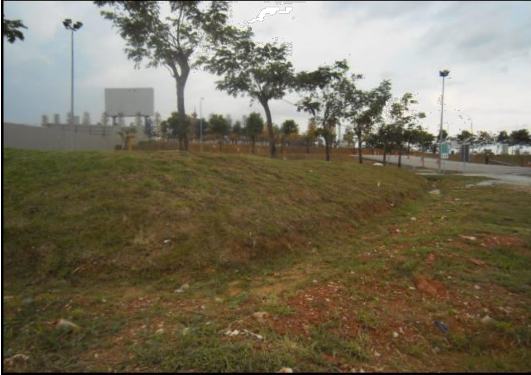
All exposed ground, slopes are turfed
