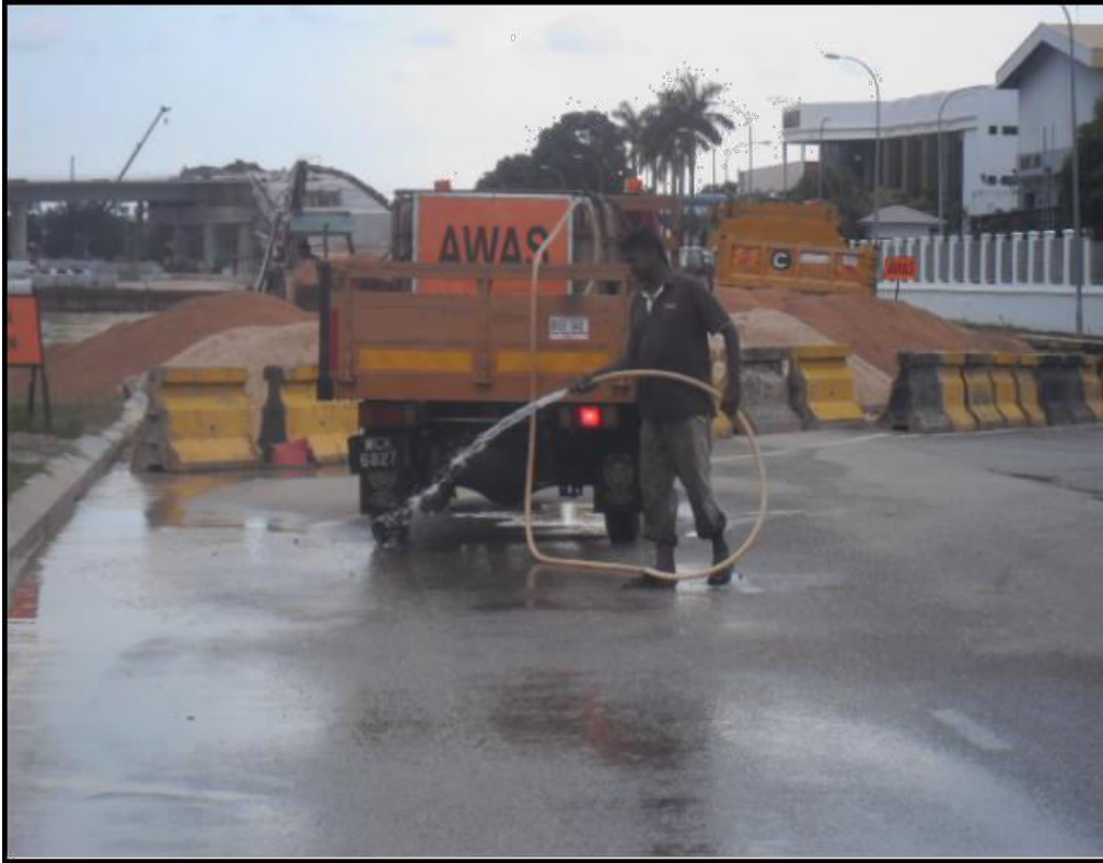
Road watering at truck trails
