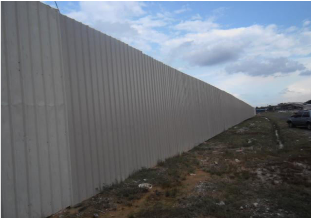
12ft high perimeter fencing provided at site
