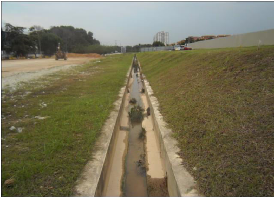
Cemented and cascade drain
