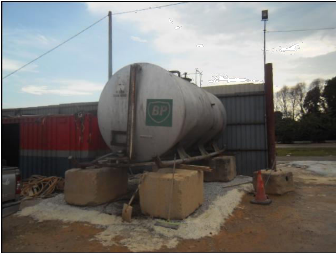
Waste oil contained in demarcated area
