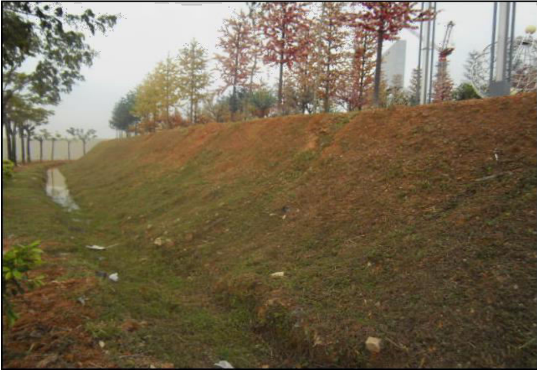
Exposed slope turfed
