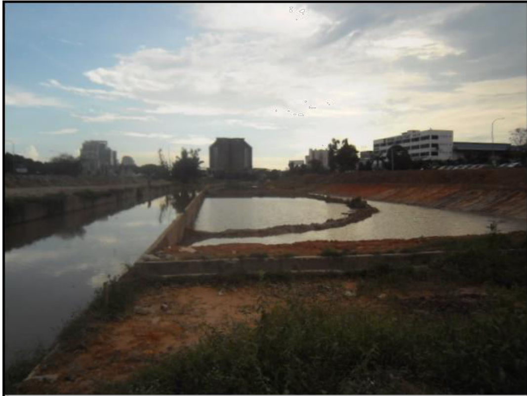
Sediment basins provided next to Sg. Rasau
